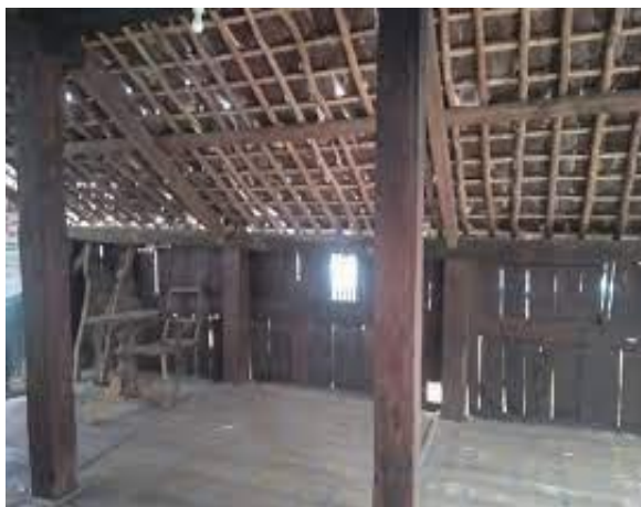
Figure 3. The interior of the Panjalin traditional house
