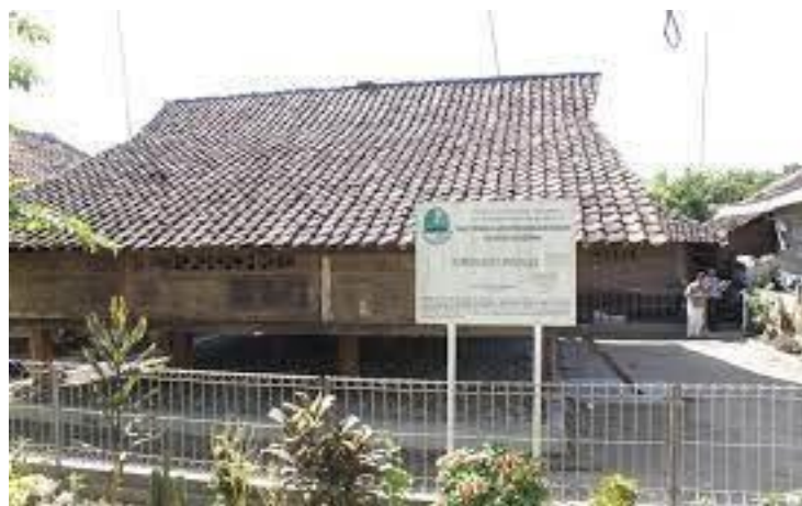
Figure 2. Panjalin traditional house
